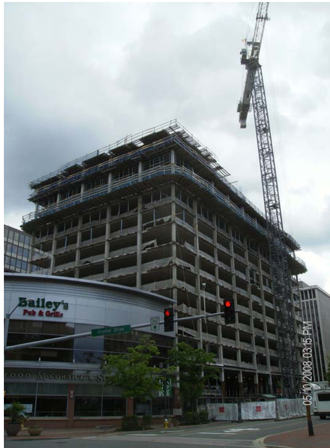
Figure 20 Superstructure and facade phase beginning
