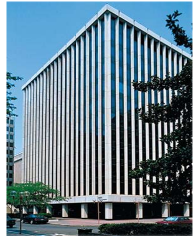
Figure 9 Existing precast façade to be removed
