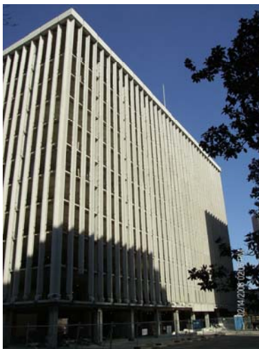
Figure 4 Exterior precast façade, south, to be removed
