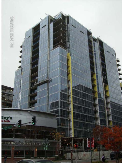
Figure 16 Stored and installed curtain wall panels
