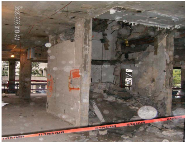
Figure 14 Demo of existing stair tower
