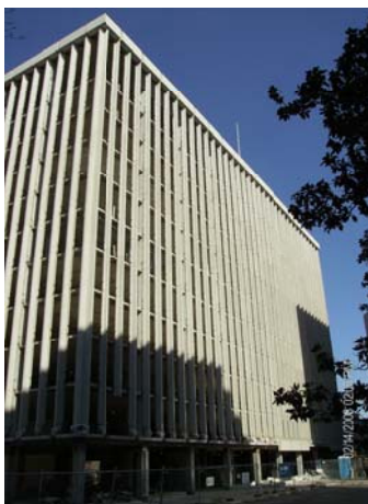
Figure 17 Exterior pre-cast facade to be removed
