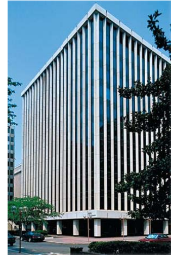
Figure 3 220 20th Street original office complex, southwest
