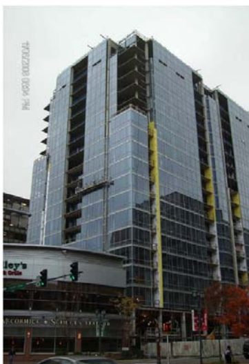
Figure 7 Installed curtain wall, northeast
